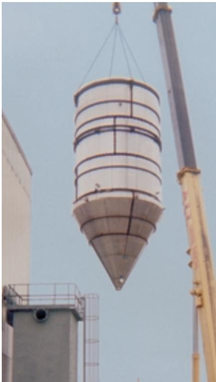
This dryer designed for centrifugal atomization awaits installation at the plant site.
