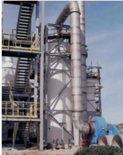
A packed bed condenser recoups energy by cooling and condensing water evaporated in the spray dryer to heat process water needed in the facility.
